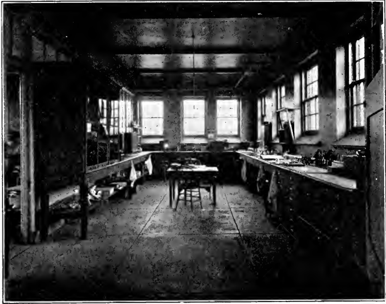
FIG. 2. GENERAL LABORATORY WORK-ROOM.
